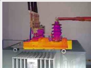
THERMAL IMAGE WITH THRESHOLD + REAL IMAGE
