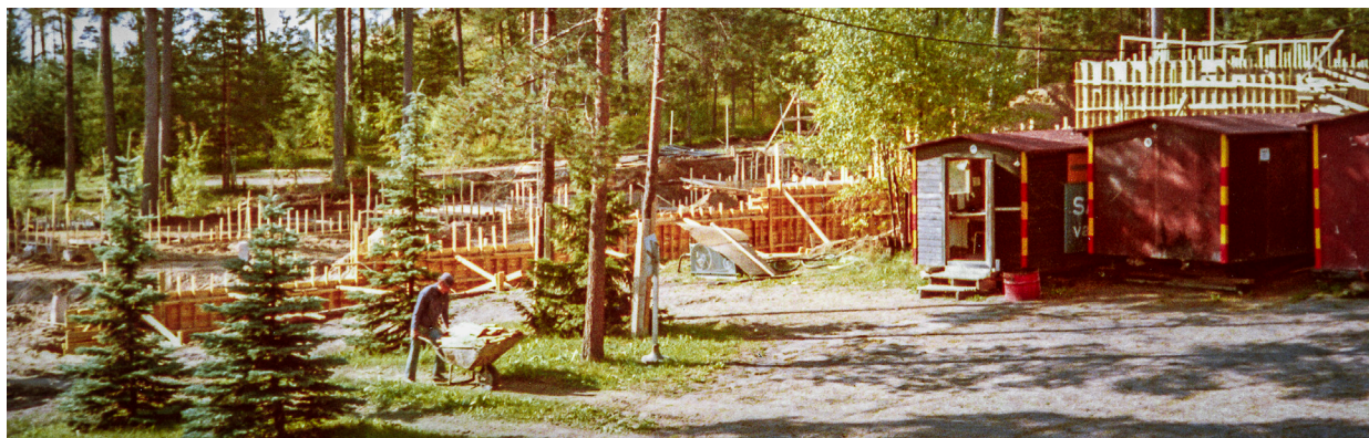
The construction of the new wing for the factory.
